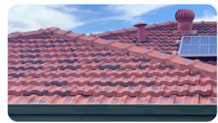
Roof Tiles Restored
