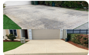
Exposed Aggregate Restored
