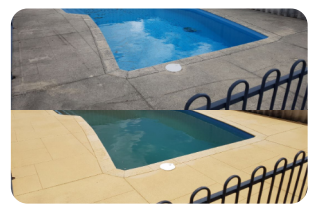
Liquid Limestone Restored
