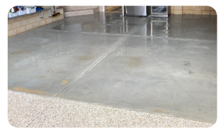
Garage Concrete Restored
